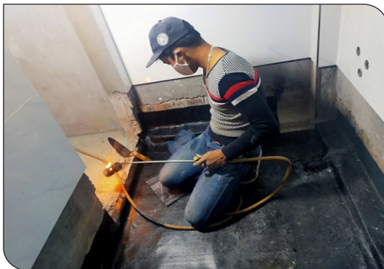
Construction of torched on membrane
